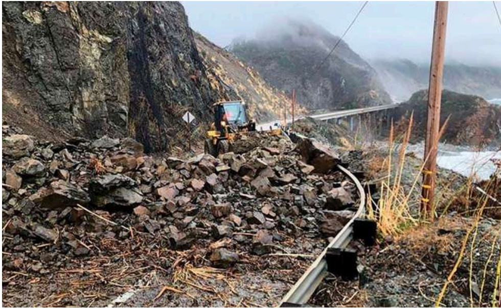
Fig: A rockslide caused by a winter storm on Dec. 7 in Big Sur, Calif Source :Caltrans.com
