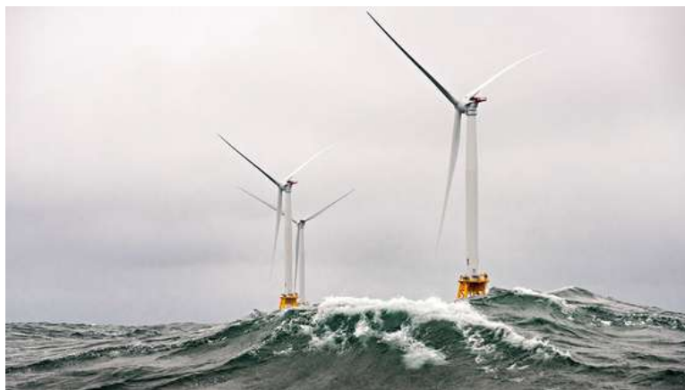
Fig: An Offshore wind Farm
