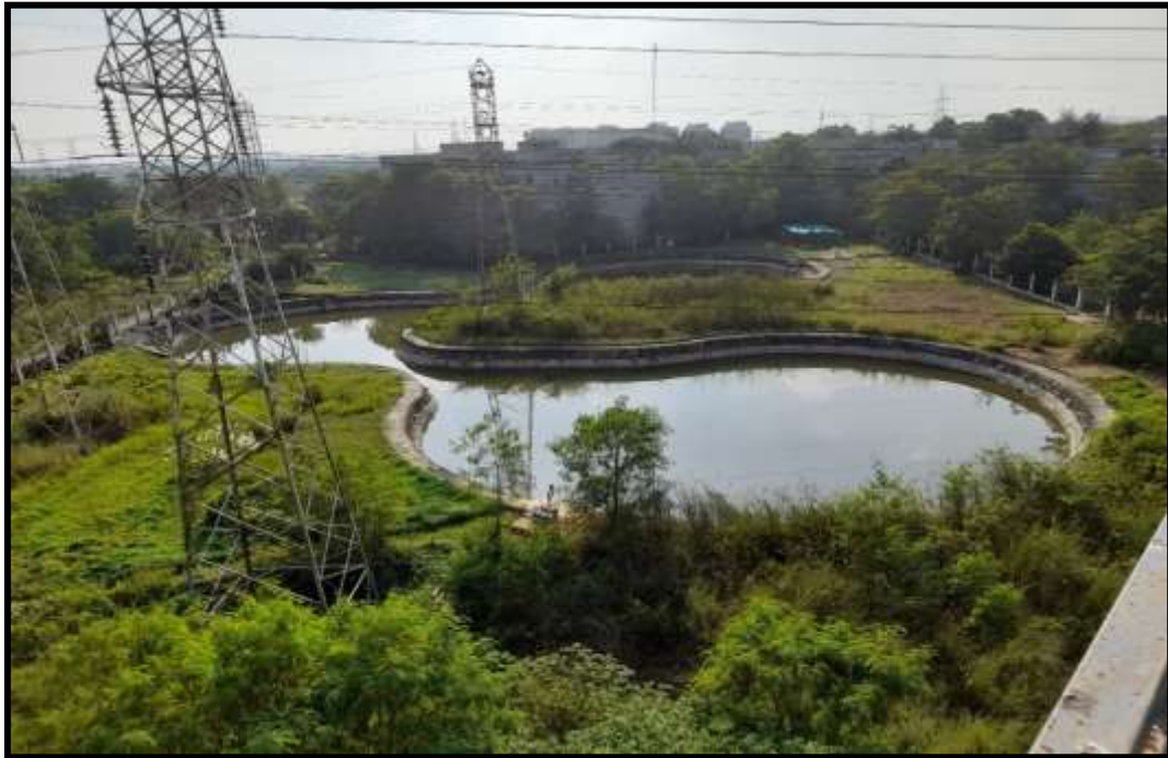
Photograph showing Rain Water harvesting pond
