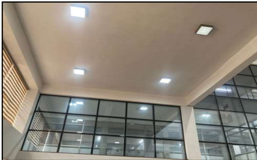
LED Lights installed in Library Block
