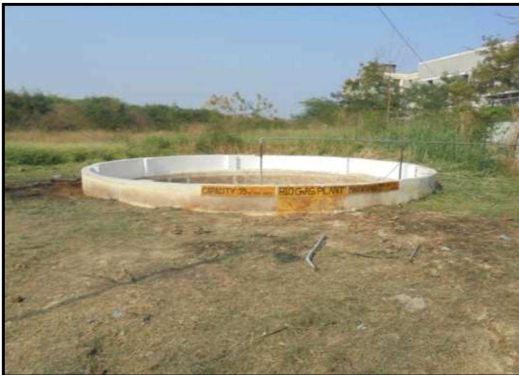
Bio Gas Plant
