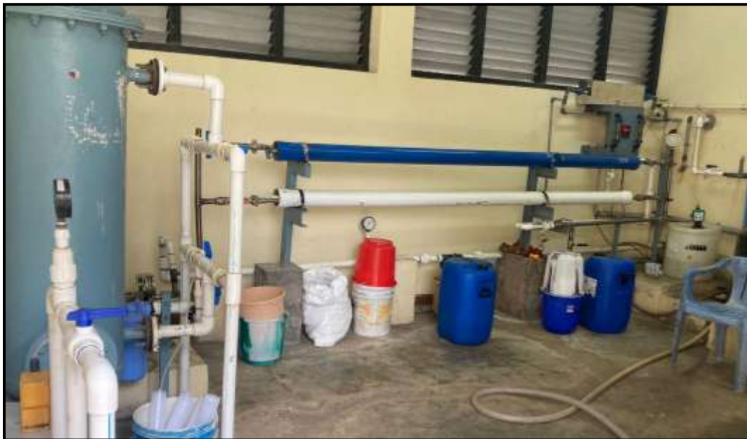
Photographs showing Water Treatment Plant
