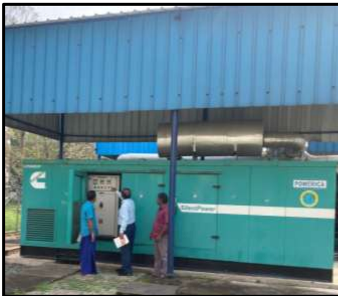
Photographs showing Diesel Generator with Acoustic enclosure & Stack Arrangements
