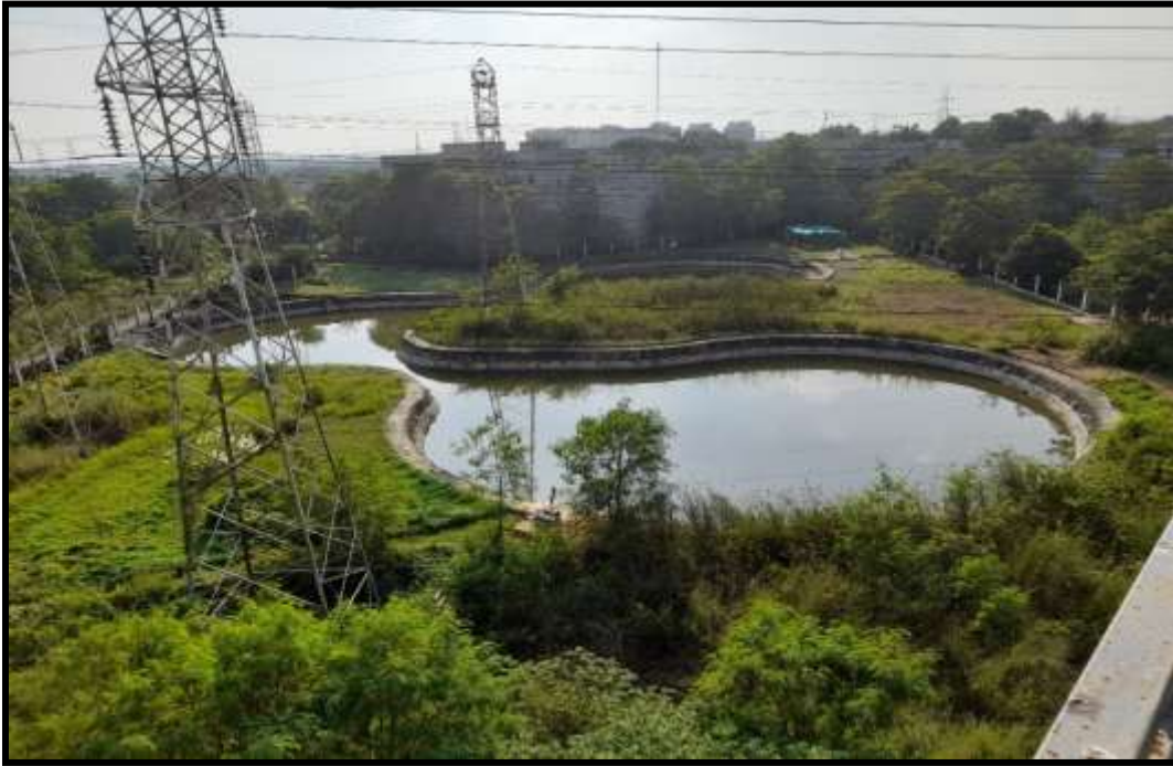
Photograph showing Rain Water harvesting pond
