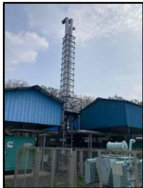
Photographs showing Diesel Generator with Acoustic enclosure & Stack Arrangements
