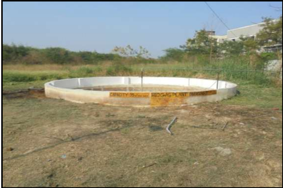
Bio Gas Plant
